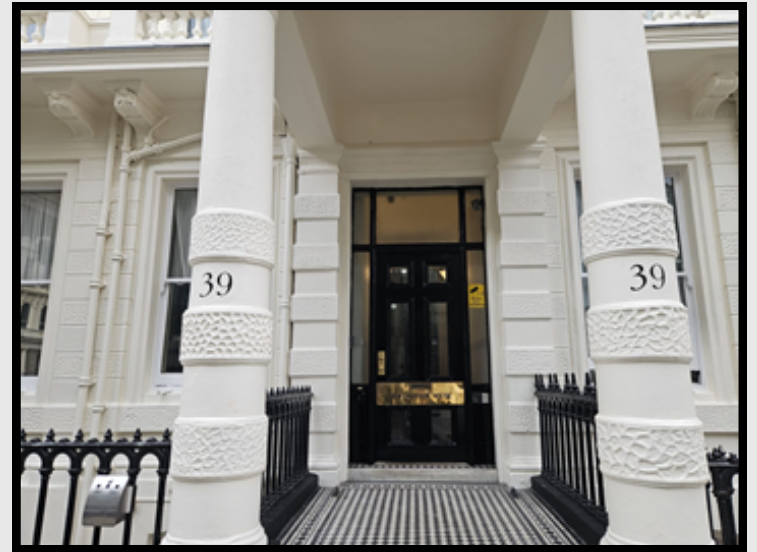
New Mansion - External Refurbishment
