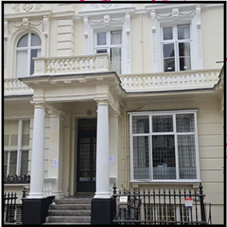
Sandeman-Allen - External Refurbishment
